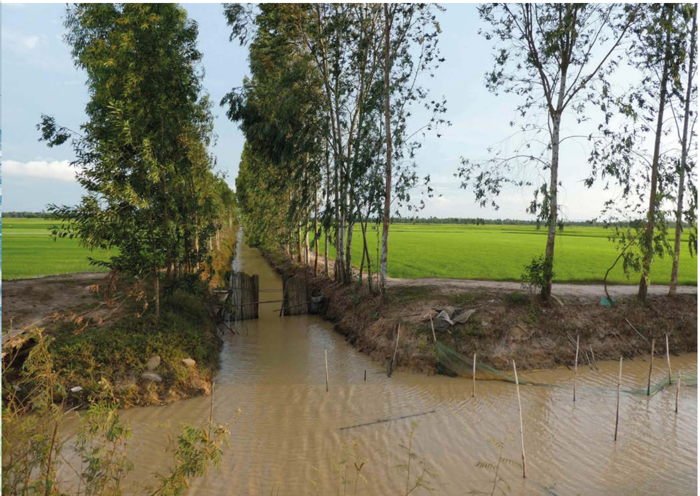
Irrigation system in the Mekong delta, Cambodia © Jean-Philippe Venot
