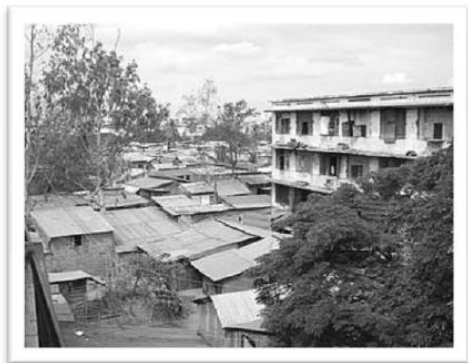
Original apartment blocks, built for athletes in 1966, now crumbling and surrounded by shacks (Author's photo, January 2006)
