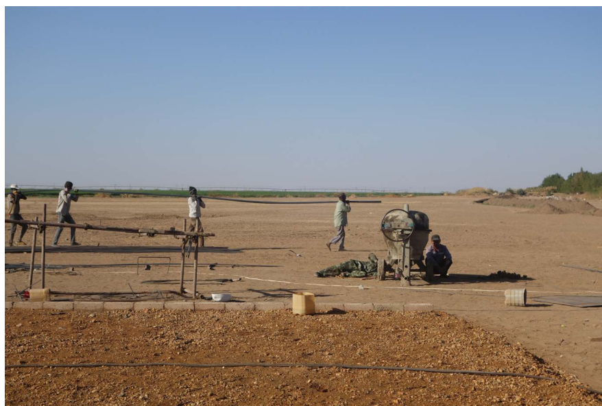
Figure 10.6 Construction site of the new ginning factory, Green Wall Company.
